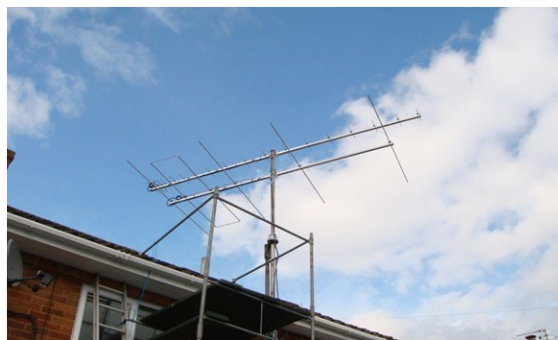
New rotator and bearing fitted then 432/70MHz fitted on mast
